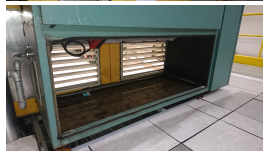
AC unit next to PT barracks.
