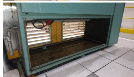
AC unit next to PT barracks.
