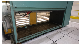
AC unit next to PT barracks.
