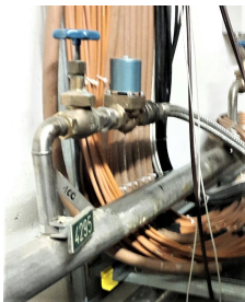
Water leak in the tunnel.
