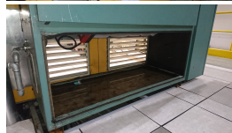
AC unit next to PT barracks.
